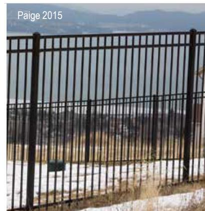
Above: A solid top rail and narrow vertical bars on this iron fence reduce hazards to wildlife.
